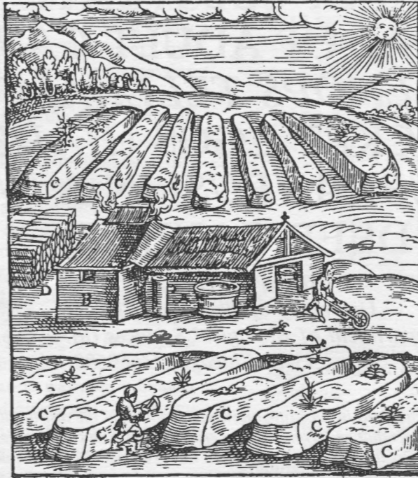
[FIGURE 41.—A SALTPETER WORKS, WITH BEDS AND BOILING-HOUSE]
